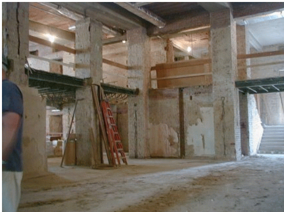
Auditorium existing atrium, under construction
