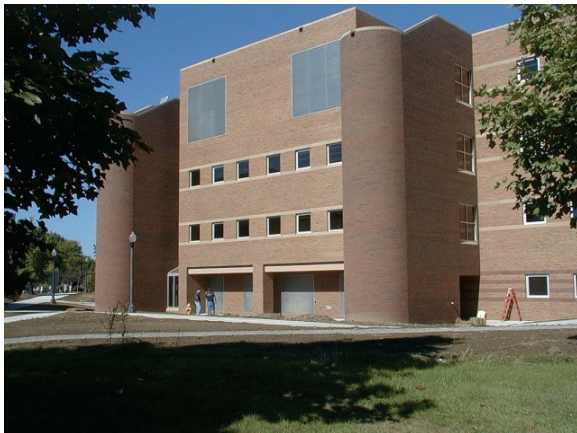
Addition to Cunningham Hall, Exterior
