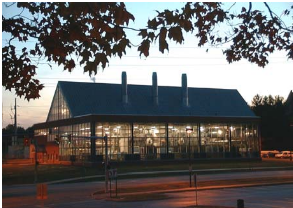
Power Plant, Exterior
