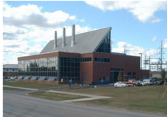
Power Plant, Exterior
